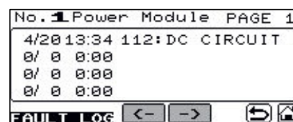
Figure 19 Power Converter Failure Log
